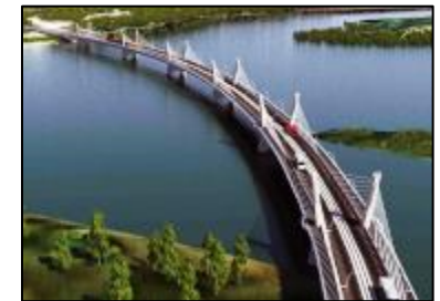
Kazungula Bridge Project (Officially opened on May 11, 2021)
