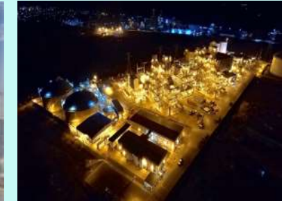
Kpone Power plant in Ghana (340MW)
