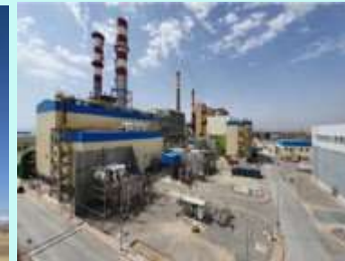
Rades-C Power plant in Tunisia (450MW)
